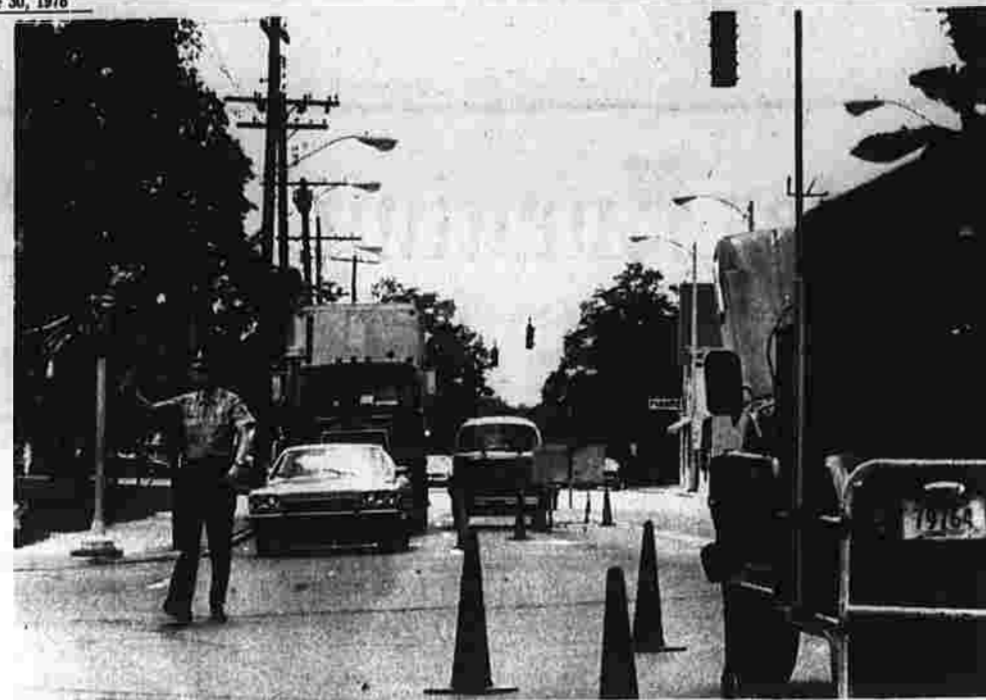
Removing old SNET connections
